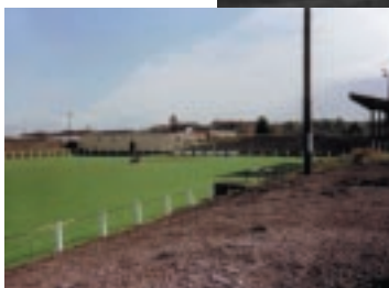
Photograph of football stadium where COPR has been used in order to form terracing for spectators.
